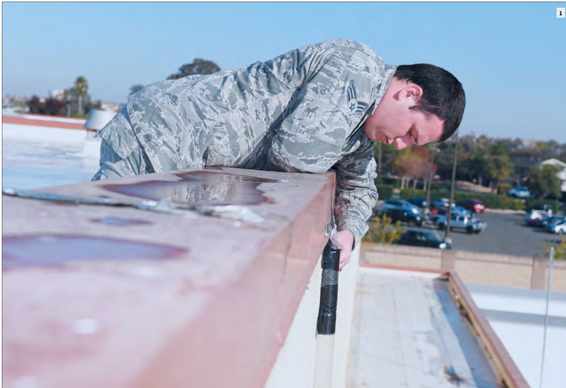
1) Senior Airman David De Alva, 60th Civil Engineer Squadron pest management technician, checks traps to see if there is any evidence of bats crawling through the pipes Nov. 8 at Travis Air Force Base, California. De Alva is trying to rid a building of bats by waiting for them to leave and blocking all entrances before they return. 2) De Alva puts on his gas mask to check if the filters are working properly Nov. 8 at Travis. 3) De Alva sets down a trap to catch vermin Nov. 8 at Travis. De Alva places traps around the base to capture unwelcome critters.
